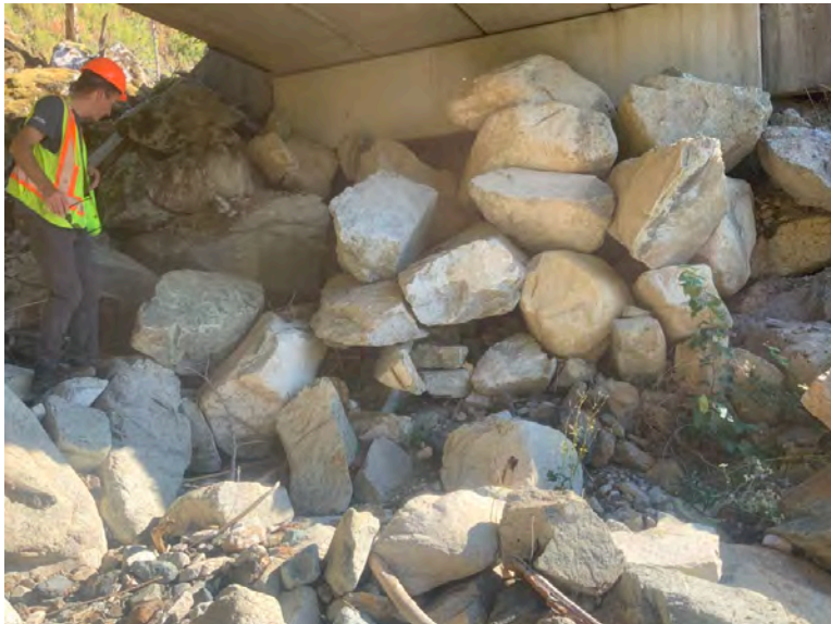
Left Bank Abutment when facing downstream
