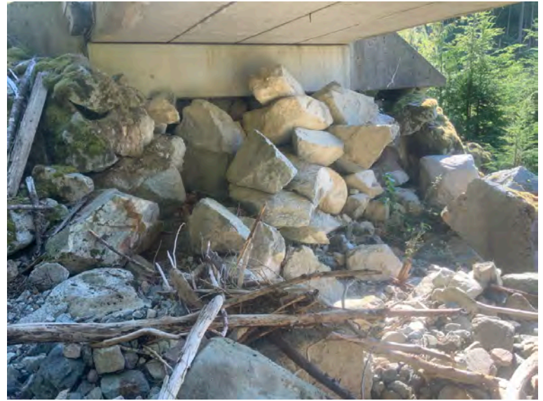
Left Bank Abutment when facing downstream
