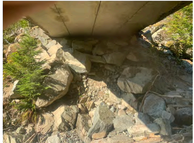
Right Bank Abutment when facing downstream
